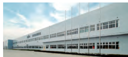
Fujitsu General Central Air-conditioner (Wuxi) Co., Ltd. (Chiny)
